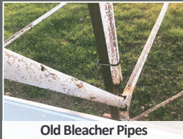
Old Bleacher Pipes
