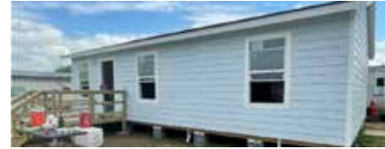
New three-bedroom, two-bathroom home built by multiple volunteer groups. Major upgrade!
